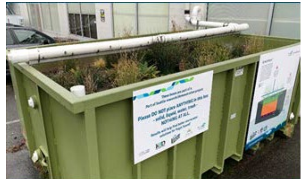
Figure 2. Splash Boxx at MIC receives roof runoff
